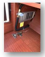
In case you need to insulate the gas inlet in the kitchen under the oven, opening the cupboard there is the gas outlet valve in the kitchen. When the valve is parallel to the pipe it is open and when it is perpendicular to the pipe it is closed.
