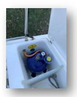
For more safety if you want to close all system of gas you need to go outside at the starboard side and to open the locker. There, you will find the bottle gas. If you turn the valve clockwise you open the gas system and when you turn the valve from the other direction you close the gas system.
