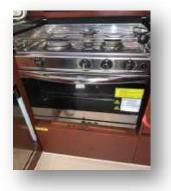
In order to turn on the oven or a hob, press the respective switch inwards and turn clockwise. Without letting go light up the hob with a lighter and hold for 5 seconds, then release. If the flame does not hold try holding in the switch for longer. Also make sure no liquids are spilled on the hobs.
