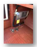
In case you need to insulate the gas inlet in the kitchen under the oven, opening the cupboard there is the gas outlet valve in the kitchen. When the valve is parallel to the pipe it is open and when it is perpendicular to the pipe it is closed.
